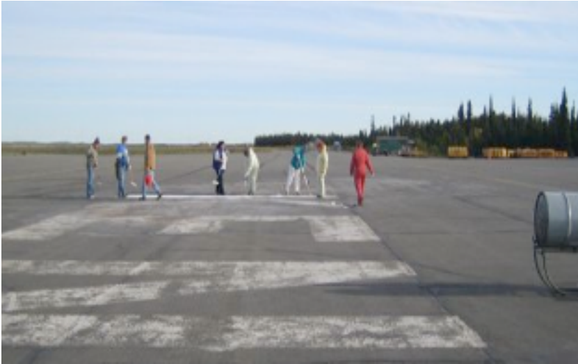
99s getting ready to start a badly needed repaint at Kenai.
